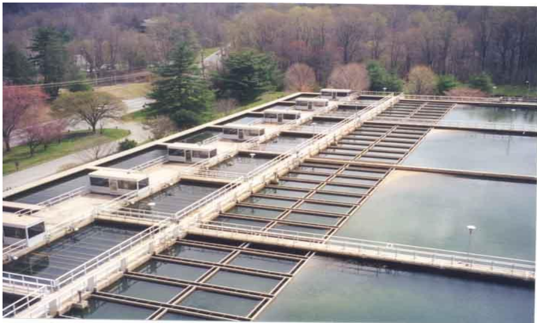
Fig: Rectangular Sedimentation Tank
