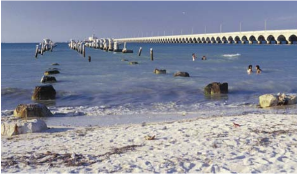
Figure 4.2 The pier on the right was built with stainless-steel rebar in Progreso, Mexico between 1938 and 1941. The remains of a parallel pier built 30 years later with black steel rebar can be seen in the foreground.
