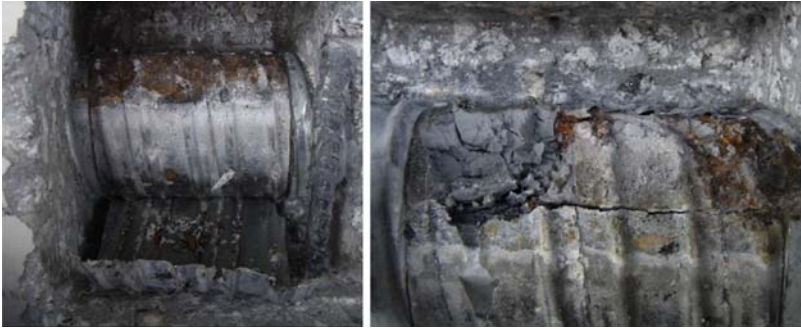
Figure 3.7 Corrosion of metal duct with deficient grout. Photos courtesy of Florida Department of Transportation.
