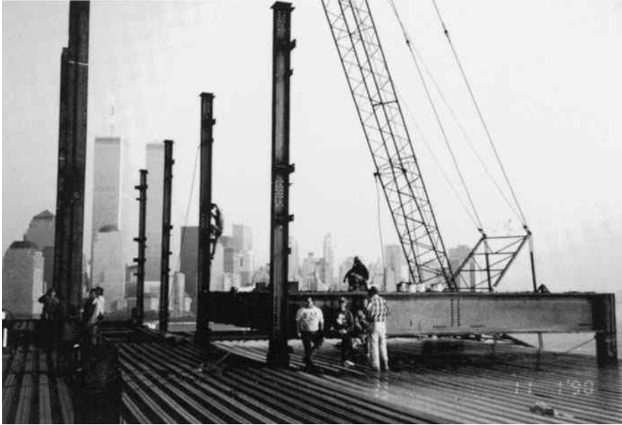
101 Hudson St., Jersey City, NJ. (Courtesy of Owen Steel Company, Inc.)
