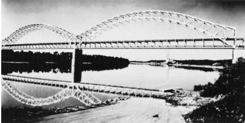
New Albany Bridge crossing the Ohio River between Louisville, KY, and New Albany, IN. (Courtesy of the Lincoln Electric Company.)
