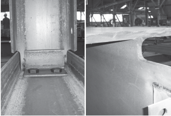
The beam on the right has a coped top flange, while the beam on the left has both flanges coped because its depth is very close to that of the supporting girder. (Courtesy of CMC South Carolina Steel.)
