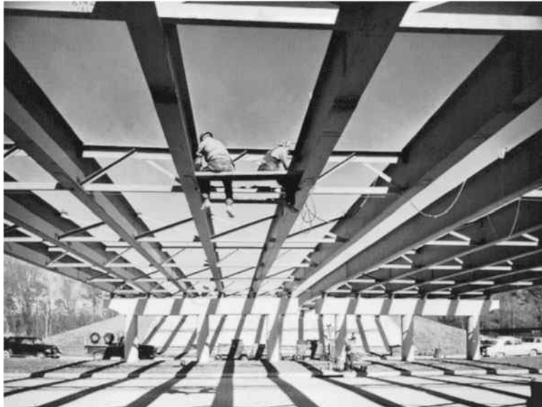
Harrison Avenue Bridge, Beaumont, TX. (Courtesy of Bethlehem Steel Corporation.)
