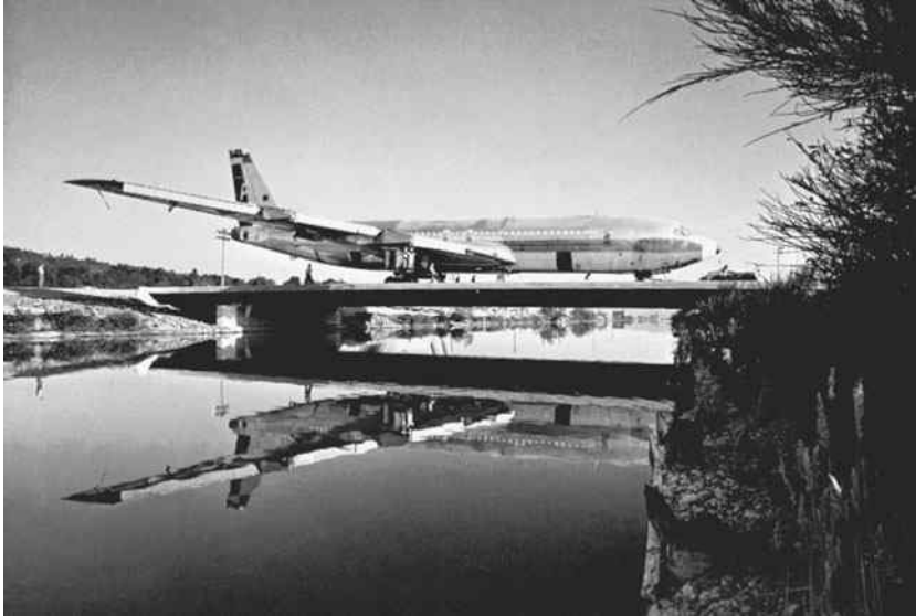
Access bridge, Renton, WA. (Courtesy of the Bethlehem Steel Corporation.)
