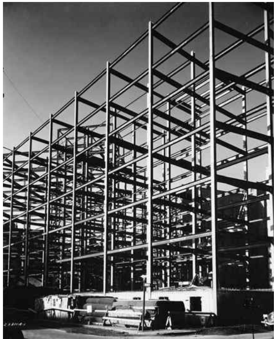
A building framework under construction. (Courtesy of Bethlehem Steel Corporation.)
