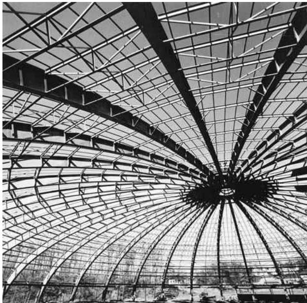
Steel dome. (Courtesy of Trade ARBED.)
