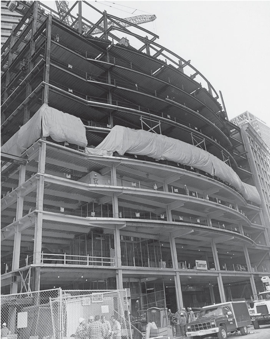
150 Federal Street, Boston, MA. (Courtesy Owen Steel Company, Inc.)
