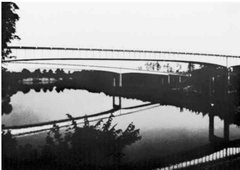
Buffalo Bayou Bridge, Houston, TX—a 270-ft span. (Courtesy of the Lincoln Electric Company.)
