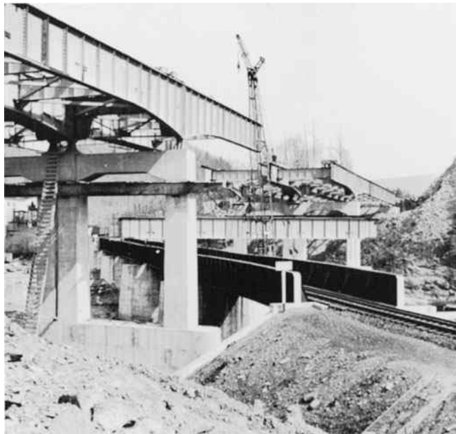
Highway bypass bridge, Stroudsburg, PA. (Courtesy of Bethlehem Steel Corporation.)
