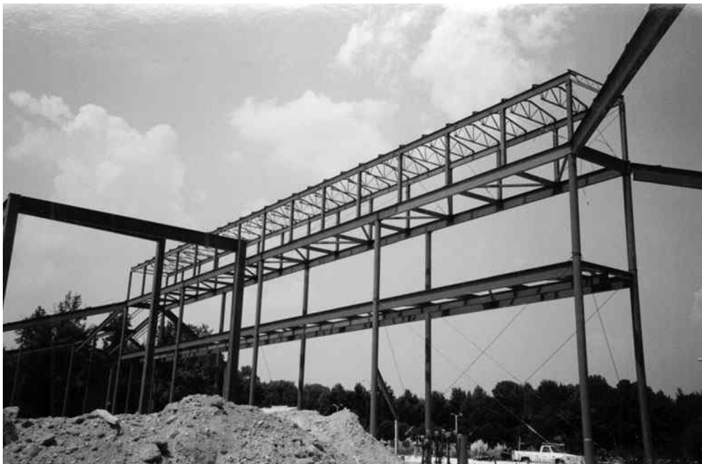
Robins Air Force Base, GA. (Courtesy Britt, Peters and Associates.)
