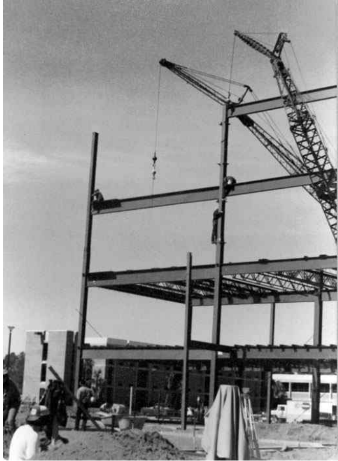
Administration Building Pensacola Christian College, FL. (Courtesy Britt, Peters and Associates.)
