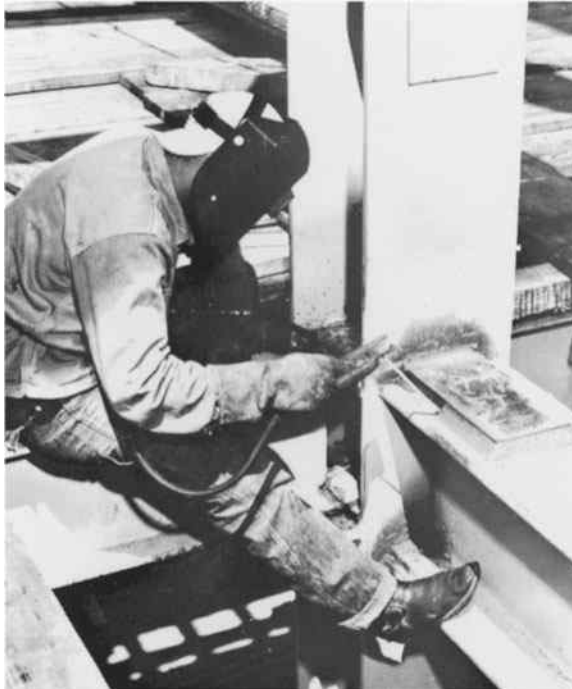
A semirigid beam-to-column connection, Ainsley Building, Miami, FL. (Courtesy of the Lincoln Electric Company.)
