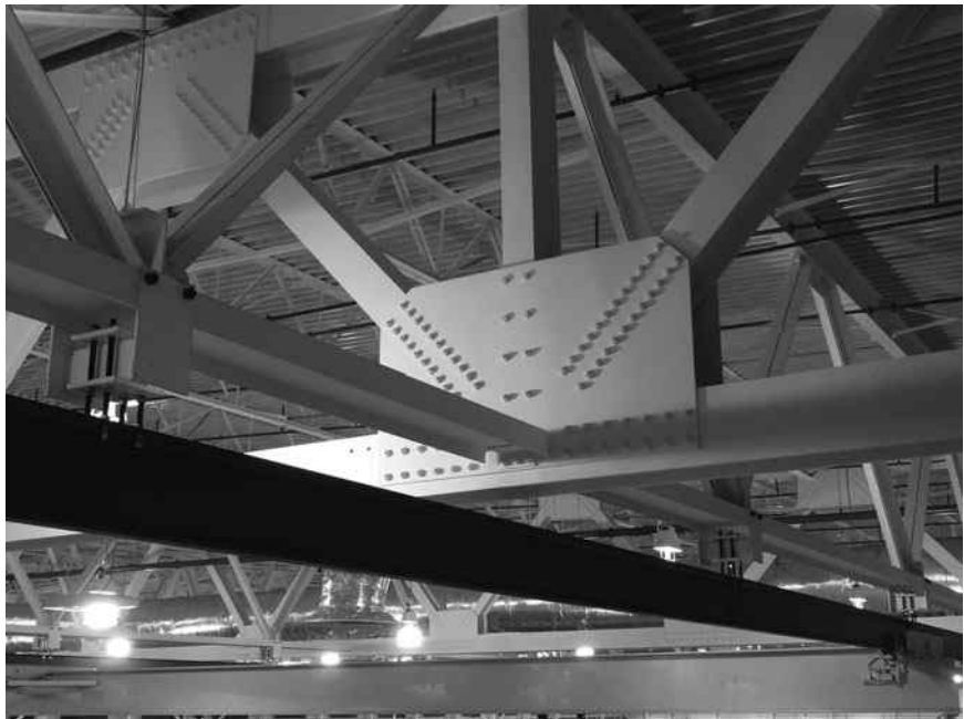
Roof/bridge crane framing, Savannah, GA. (Courtesy of CMC South Carolina Steel.)
