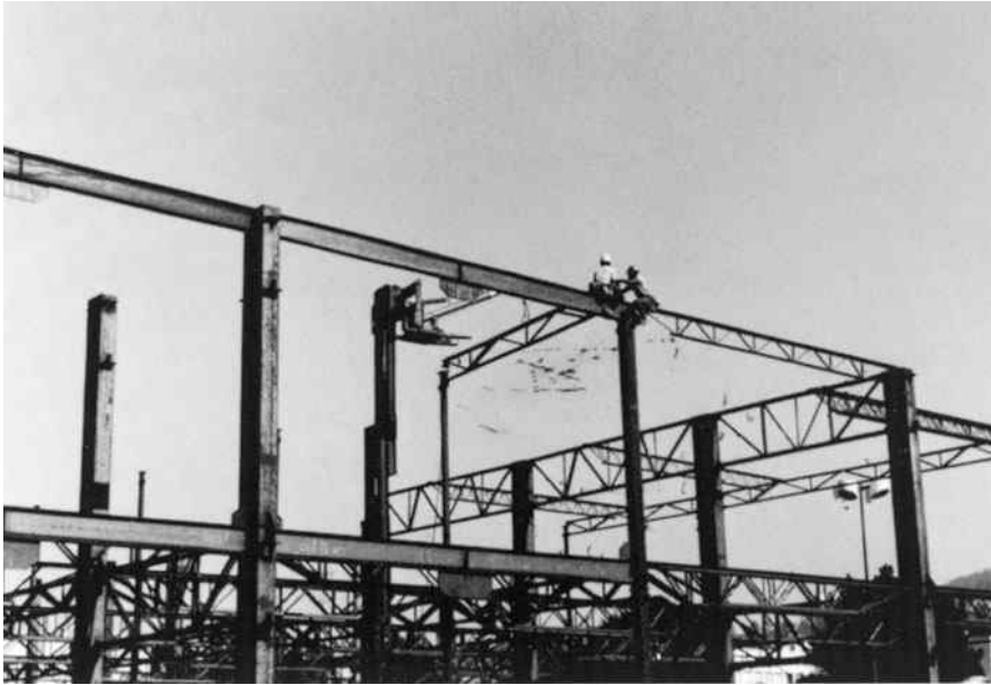
Erection of steel joists. (Courtesy of Vulcraft.)
