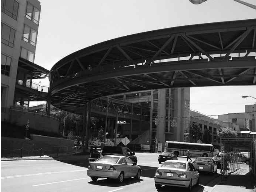
Pedestrian bridge for North Carolina Cancer Hospital, Chapel Hill, NC. (Courtesy of CMC South Carolina Steel.)
