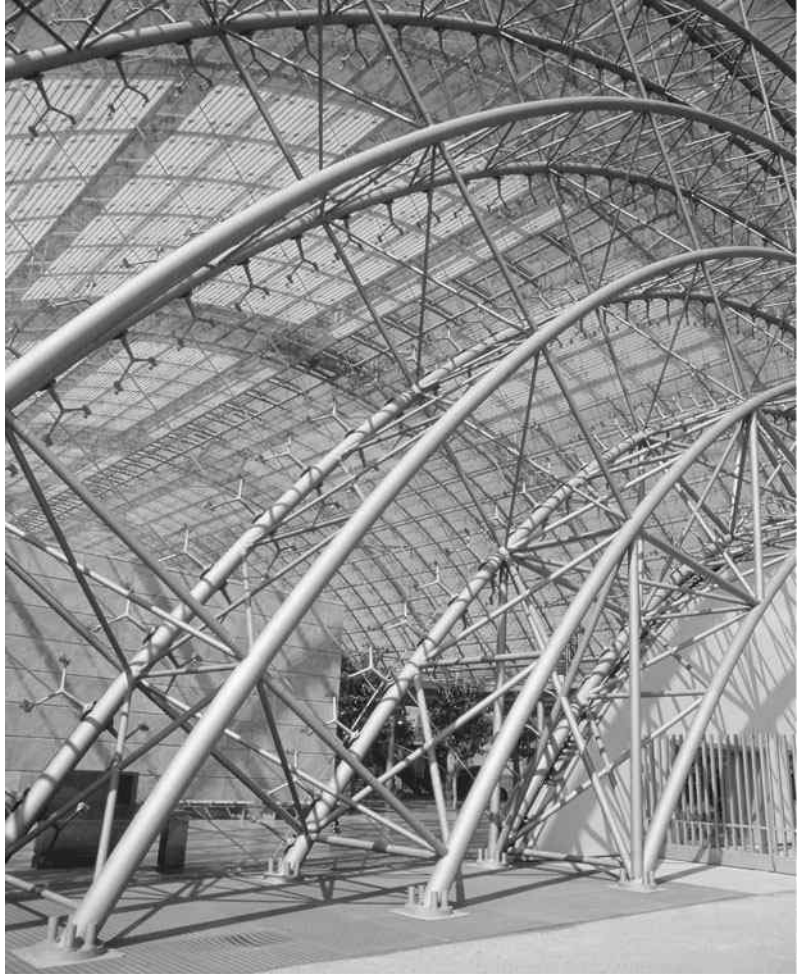
Round Arch Hall at exhibition center, Leipzig, Germany. (© Klawns Hackenberg/Zefa/Corbis. Used by permission.)
