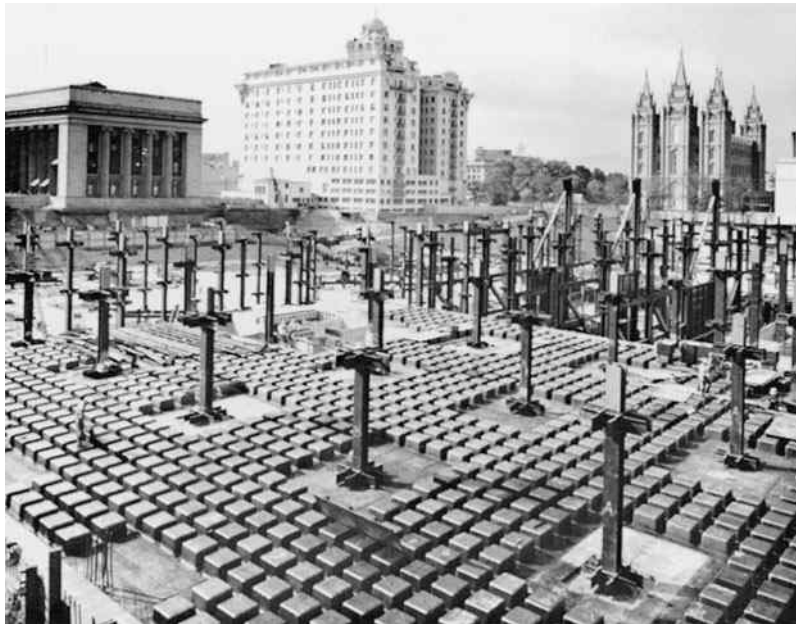
Temple Plaza parking facility, Salt Lake City, UT. (Courtesy of Ceco Steel Products Corporation.)
