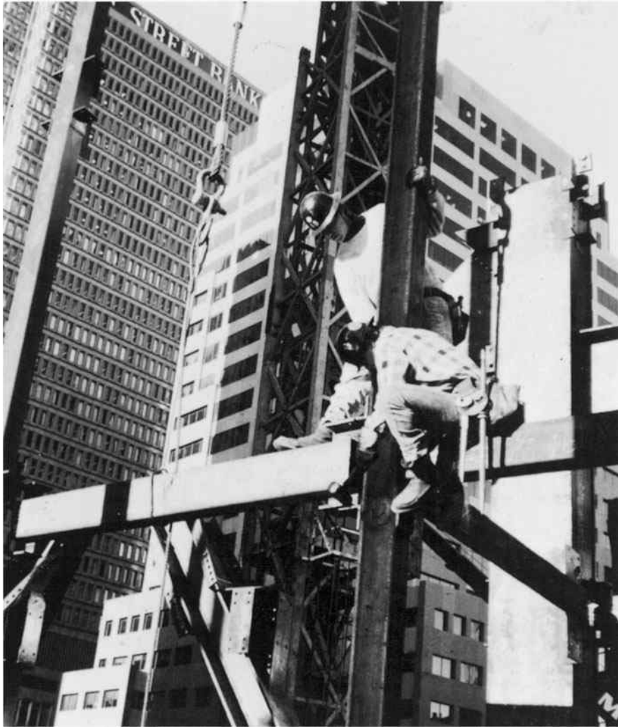
Two International Place, Boston, MA. (Courtesy of Owen Steel Company, Inc.)
