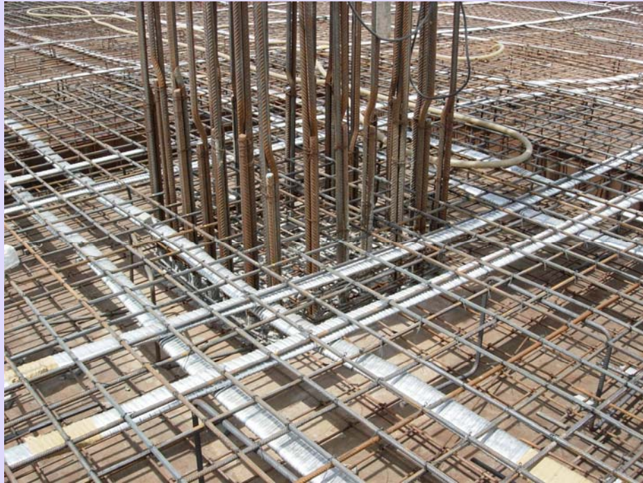
Figure 9-3.6 Reinforcement at slab-column junction (Courtesy: VSL India Pvt. Ltd.)
