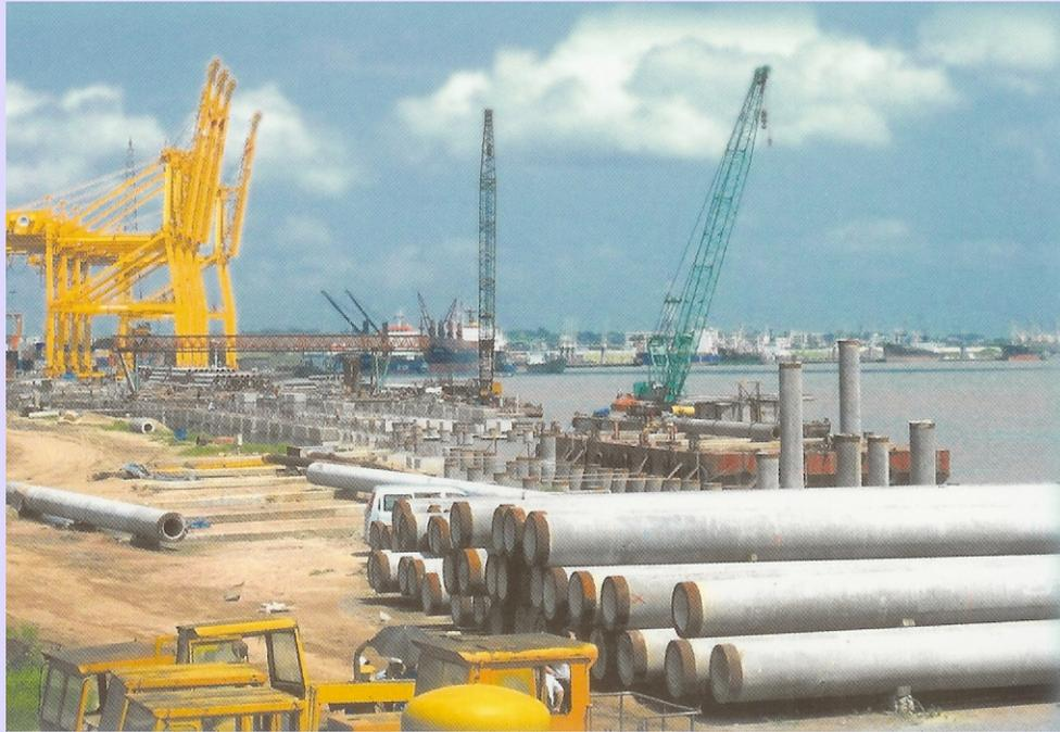
**Figure 9-5.2** Stacked prestressed piles
