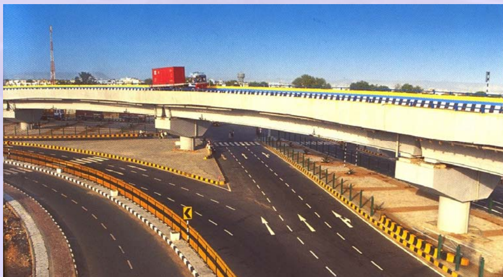
Figure 9-6.14 Curved box-girder bridge, Jaipur-Kishangarh Highway, Rajasthan (Reference: L & T Ramboll)
