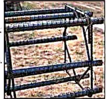
(b) Tie arrangement in a square column with 8 longitudinal bars and a set of two ties. See also (c)
