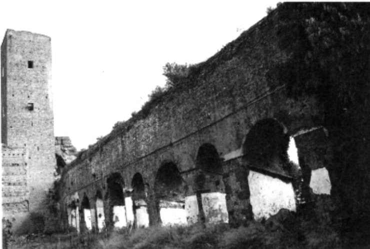
Fig. 8.1 Remains of Roman aqueduct
